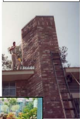
Trojan being sprayed on masonry
